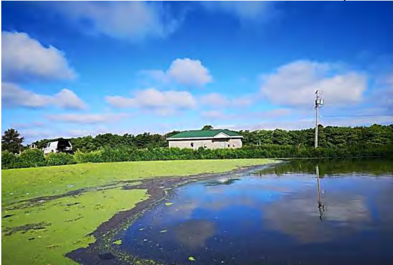
Tobermory Wastewater Biosolids Primary Retention - Cell #1.
