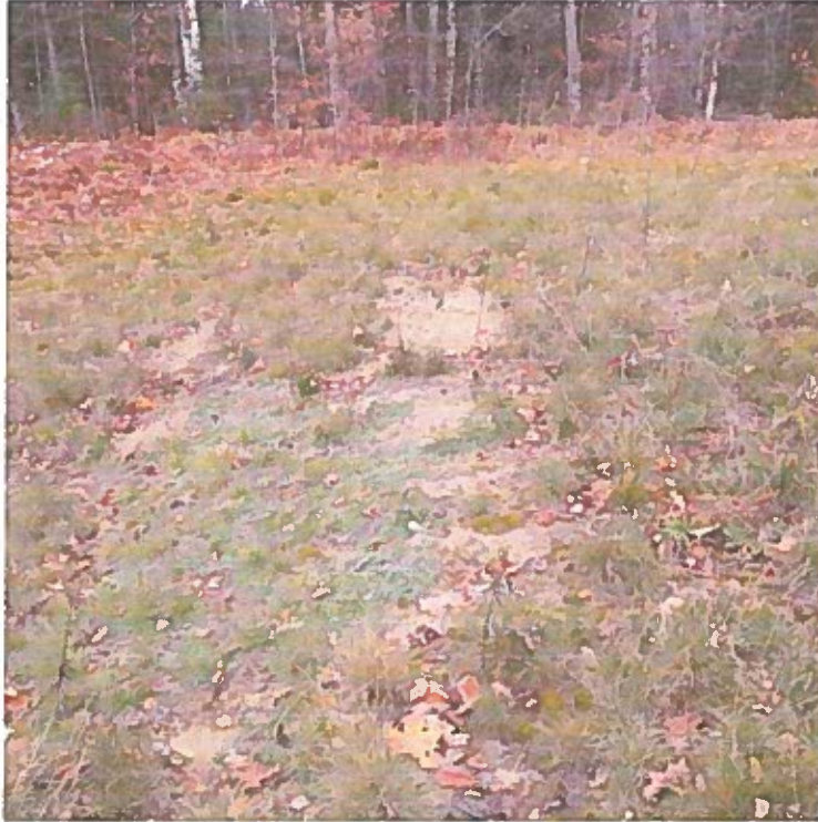
Photo ID IMG_20161114 - 125659: Topsoiling required on south slope of tile field. Southwestern corner of tile field shown in photo.
